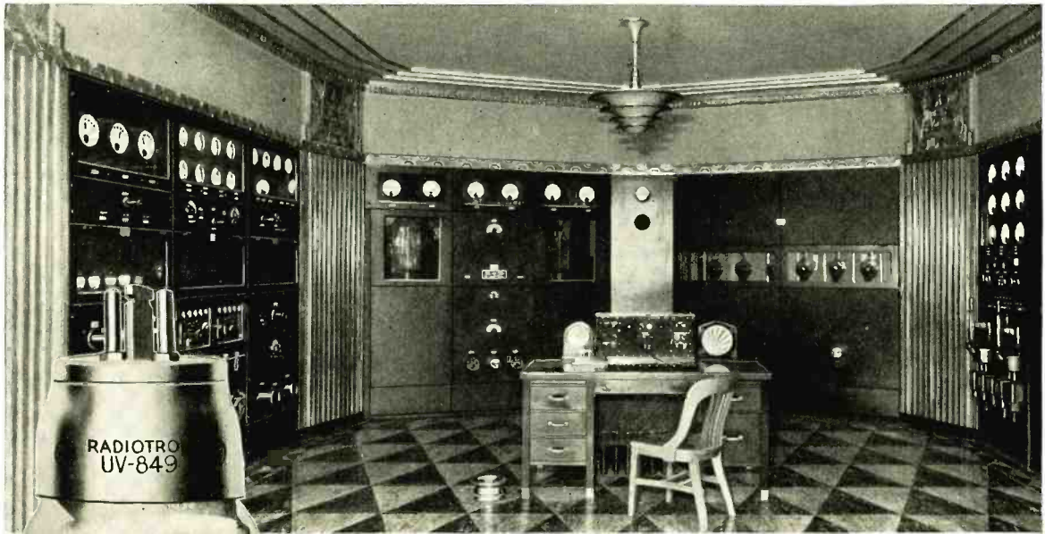
Broadcast Station WEAf—50 kilowatts
